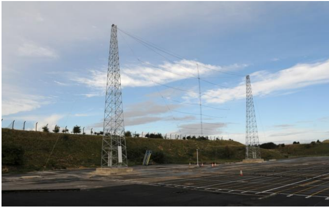
Figure 2. HF horizontal dipole antenna
